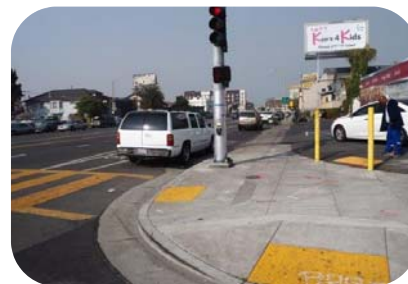
ADA ramp and signal upgrades
